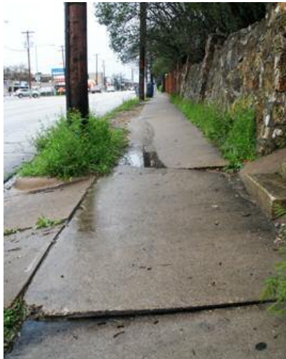
The sidewalk just north of Wheatsville is buckled and rough. It's very hard for a person in a wheelchair to navigate. It's an outrage that a major pedestrian street like Guadalupe has sidewalks that are barely usable. There are places where lightpole placement makes the sidewalk too narrow for a wheelchair. —Aldia
